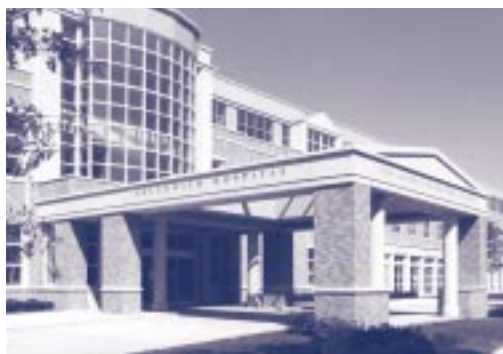
Greenwich Hospital, CT
